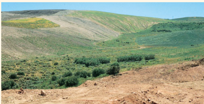
FIGURE 15.15 (a) Mining an exposed coal bed at the Trapper Mine, in Colorado; and (b) the land during restoration following mining. Topsoil (lower right) is spread prior to planting of vegetation.
