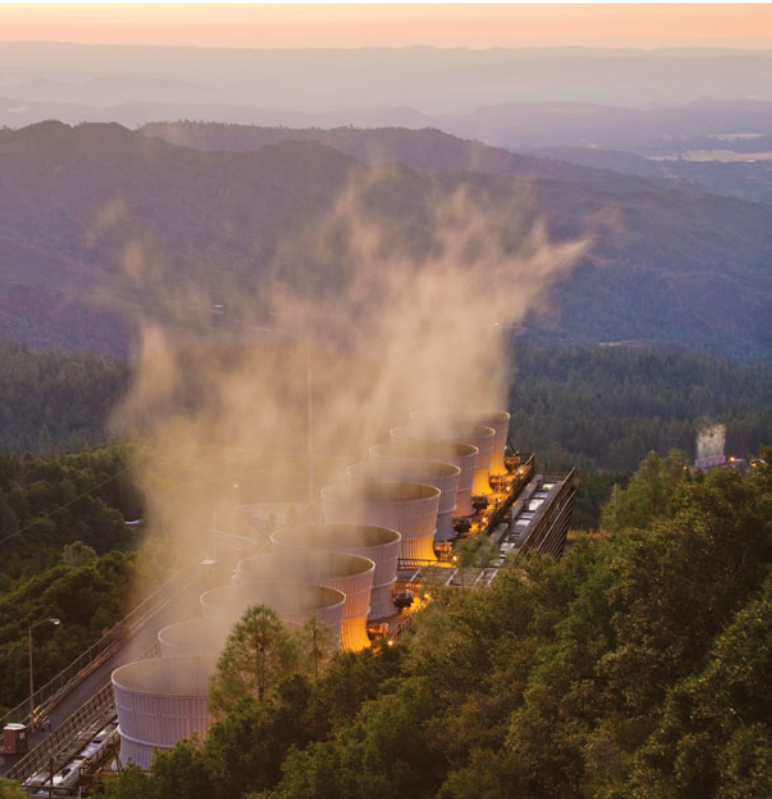
FIGURE 16.16 Geysers Geothermal Field, north of San Francisco, California, is the largest geothermal power operation in the world and produces energy directly from steam.
