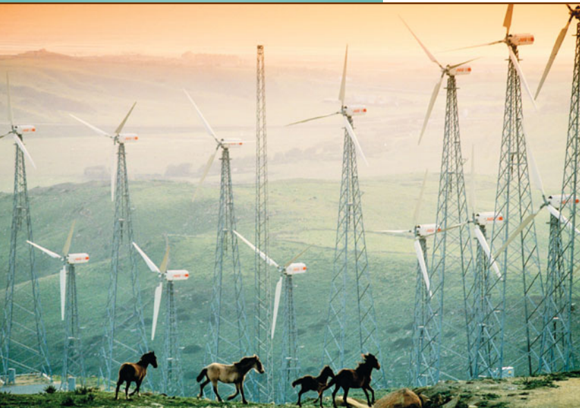
This wind farm in Tarifa, Spain, has a generating capacity of 5 MW produced by just 12 wind turbines.
