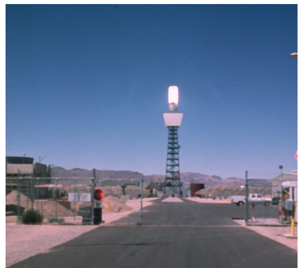
FIGURE 16.8 Solar power tower at Barstow, California. Sunlight is reflected and concentrated at the central collector, where the heat is used to produce steam to drive turbines and generate electric power. [Source: Photograph by Daniel B. Botkin.]
