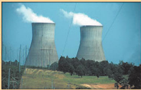
Cooling towers, Burke County, Georgia
