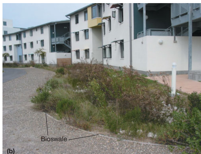
FIGURE 19.12 Bioswales collect runoff from Manzaneta Village Dormitory Complex at the University of California, Santa Barbara. (a) Plants in bioswales (b) help filter water and remove nutrients, reducing cultural eutrophication.
